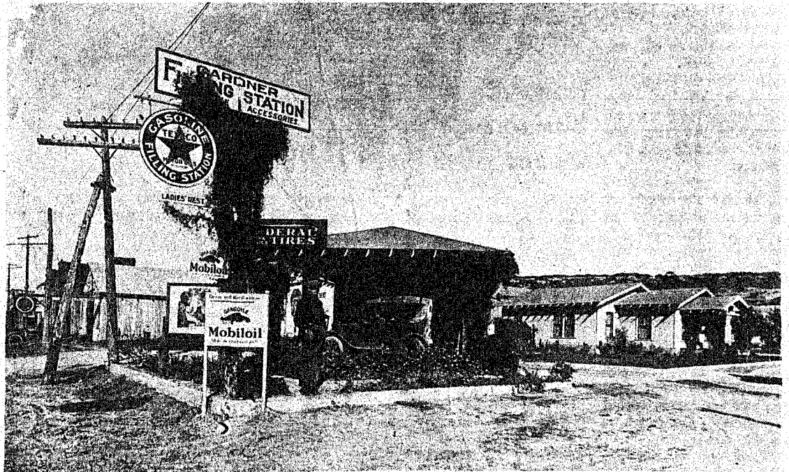
EARLY-DAY SANTA ANNA BUSINESS was Gardner Filling Station at the corner of North Lee Street and Wallis Avenue (far left). Home at right is now owned by the Tex Tomlinsons. The station featured Texaco
