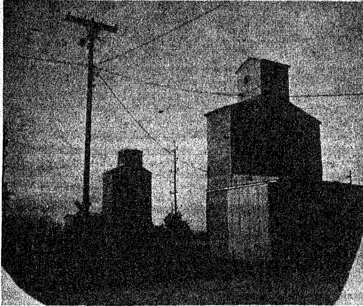
NEW OWNERSHIP of the former Santa Anna Grain Elevator was announced this week when the facility was sold to Alderman-Cave Milling and Grain Company of Winters by Terry McIver. A major renovation project is planned to begin in about a month. The facility has been in operation in Santa Anna for many years, owned originally by Santa Anna Co-Op Gin and Continental Grain Co.
