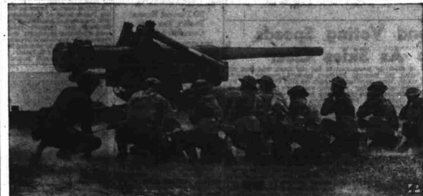
PICTURE WITH SOUND EFFECTS—Army's longest range field piece, this 155 mm. rifle speaks out at Fort Bliss. N. C. Its range is 17 miles. The gun is drawn by 175 h.p. tractor, the gun and tractor together weighing 30 tons.
