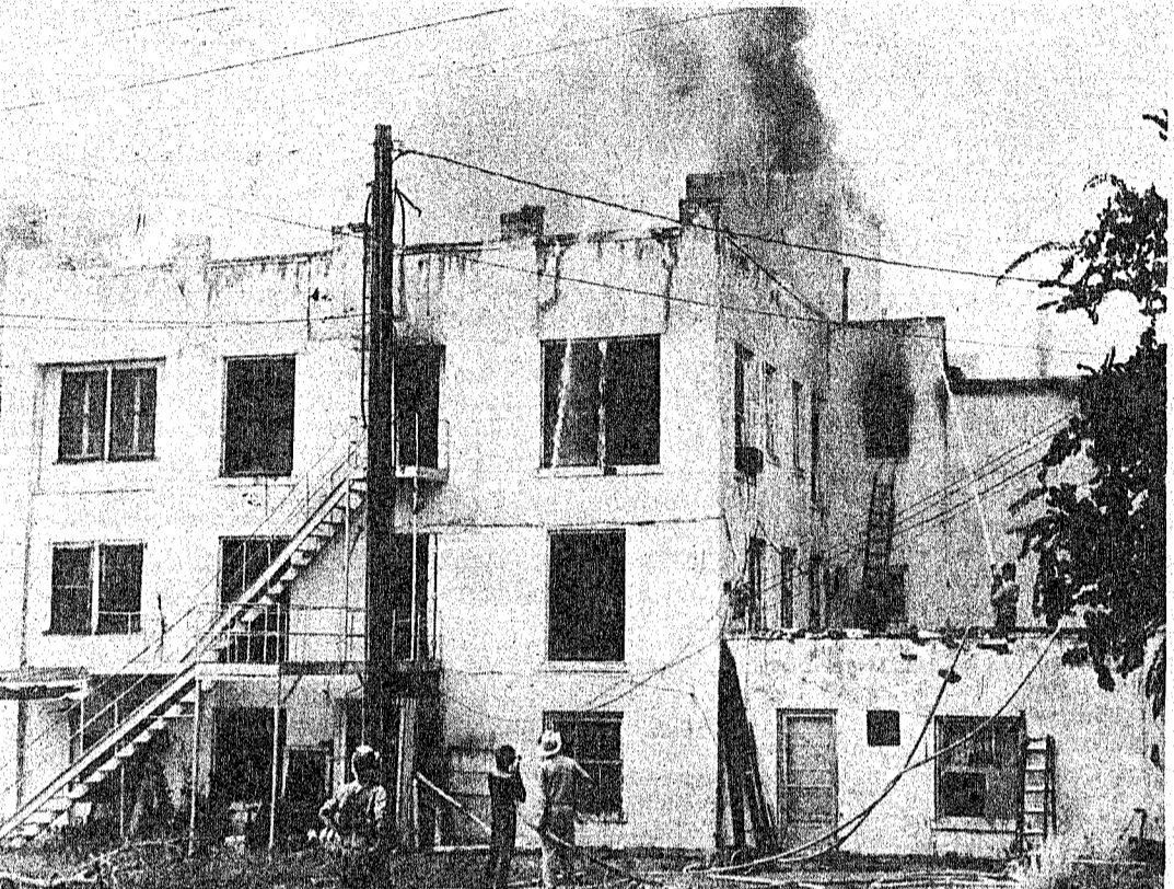
SMOKE RISES from the elevator shaft at the old Santa Anna Hospital building as the fire is brought under control Tuesday. The building is
