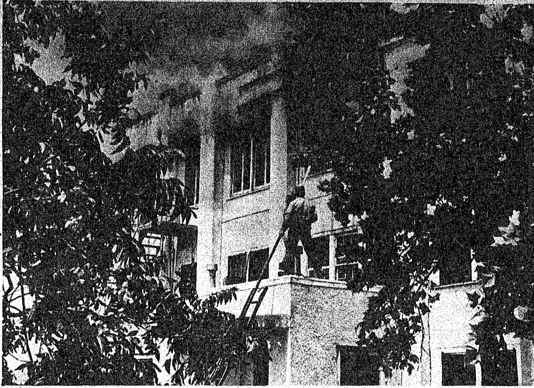
TUESDAY FIRE at the old Santa Anna Hospital gutted the upper floor and caused severe smoke and water damage to the first and second floors.
