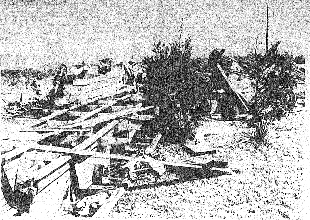
MORE DAMAGE from the June 19 storm in our community is shown here at the Roy Bell Ranch nine miles south of Santa Anna where two barns were destroyed and a mobile home torn in half. Shown here is the rubble of one barn, with the
