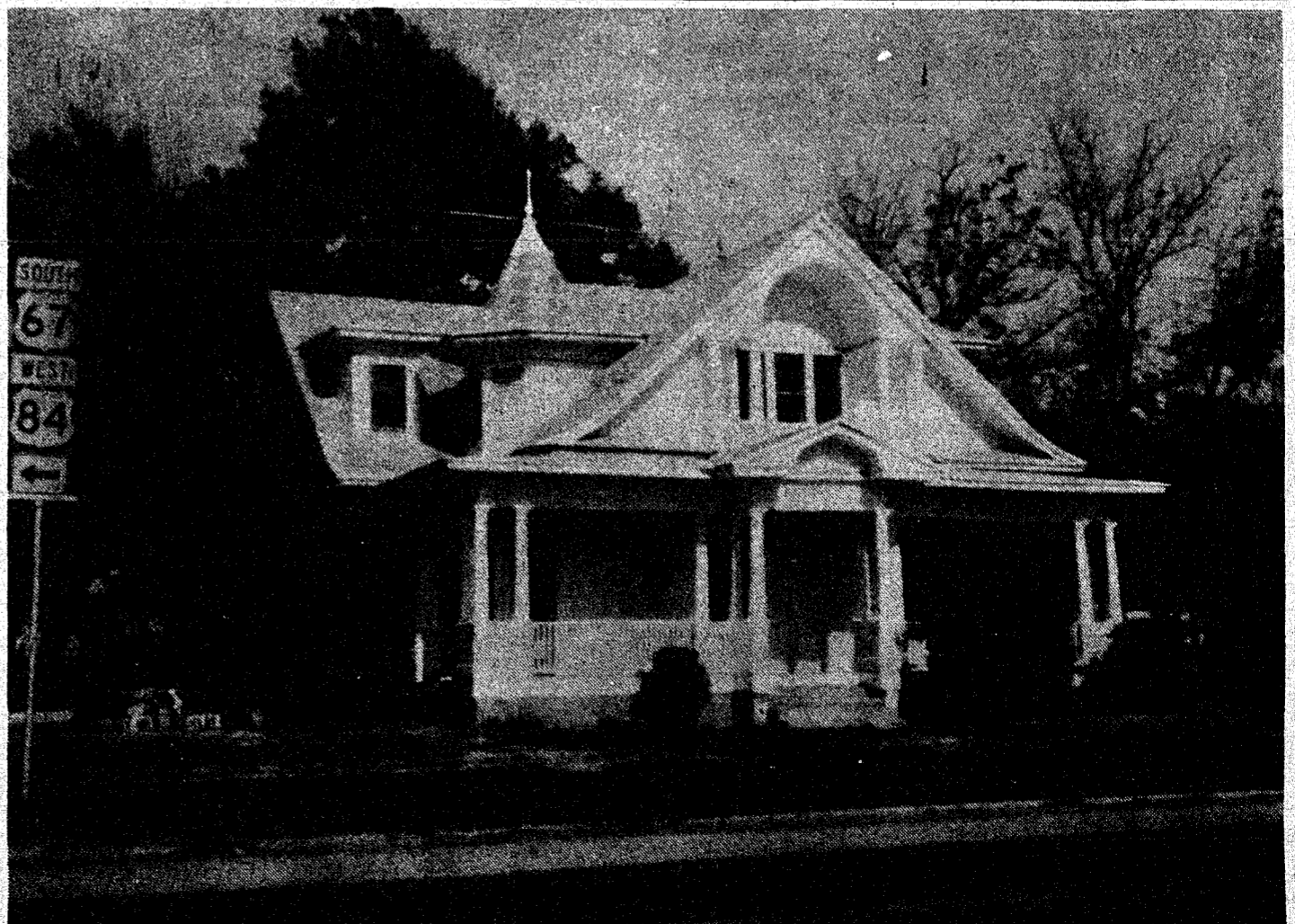
FACE LIFT..... A Santa Anna landmark has been renovated recently. The charming old home of the late Mrs. J. R. Gipson has been repainted and repaired by its present owner, Robert Stewardson. The last occupants of the
