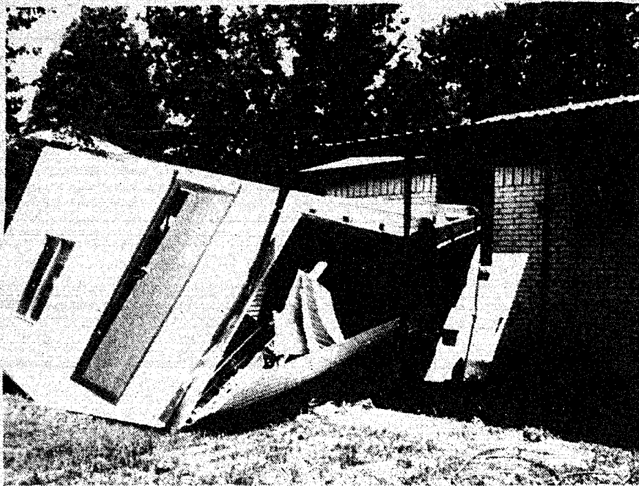
WIND DAMAGE.... A storage building at the home of Oleta Mobley on Avenue B was overturned and destroyed during the windstorm early Monday morning. Other damage was reported in town during the early morning rainstorm.
