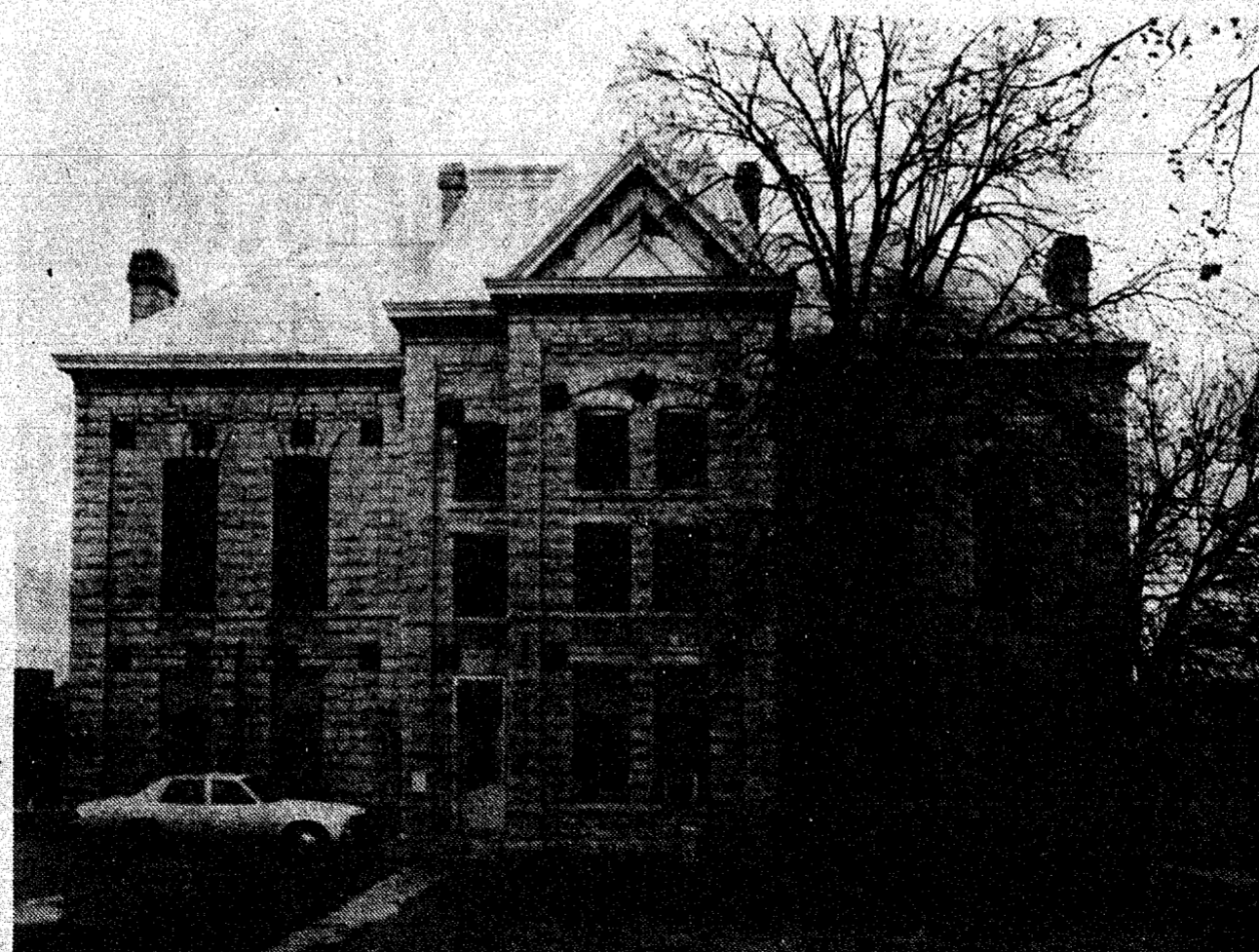
COLEMAN COUNTY JAIL— 1890 structure must be renovated to meet current jail standards or be replaced. County officials are planning improvements that are expected to cost $100,000.
