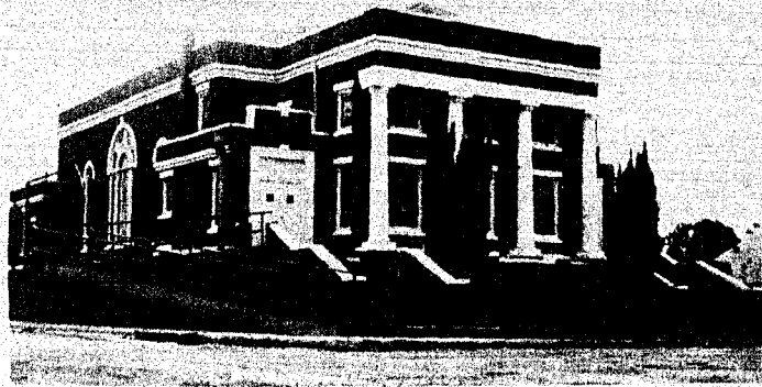
NEW RAMP at First Baptist Church has recently been completed and is in use. The ramp is of metal construction, faced with siding to coordinate with the red brick building, and covered with astro-turf carpet. Built with donations and memorial gifts, the major contributor was the Levi Smith family.
