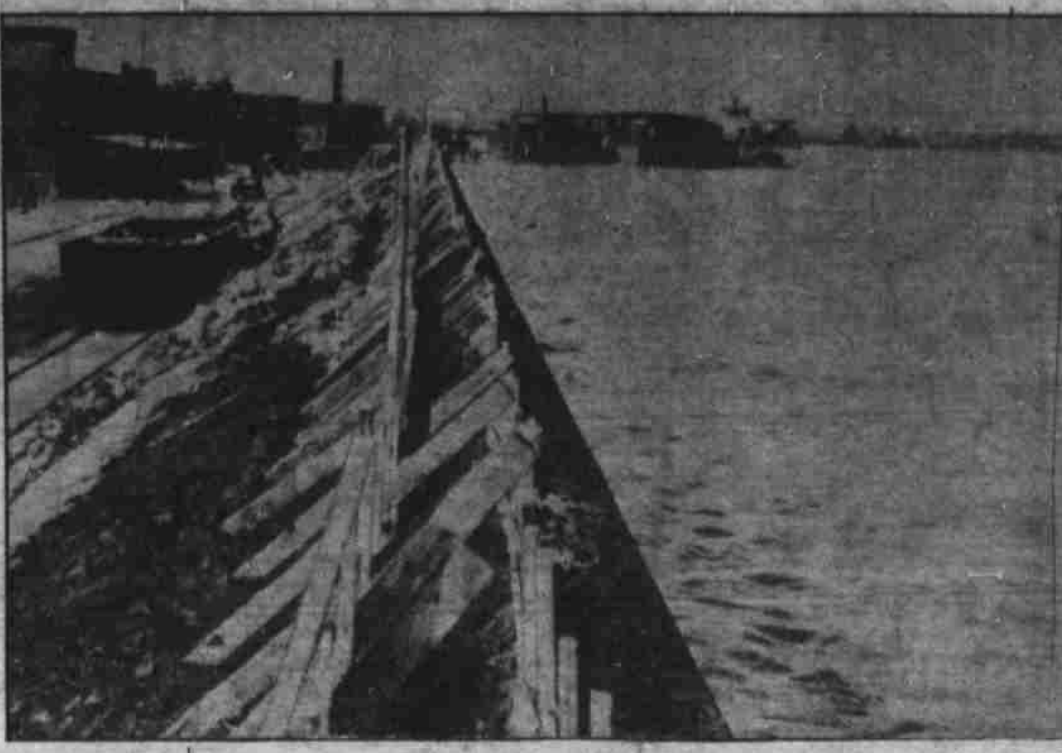
Rising flood water of the Ohio river is shown within three feet of the bulk-headed 63-foot seawall protecting Cairo, Ill. Note the water level is far above street level of the threatened town. (Associated Press Photo.)
