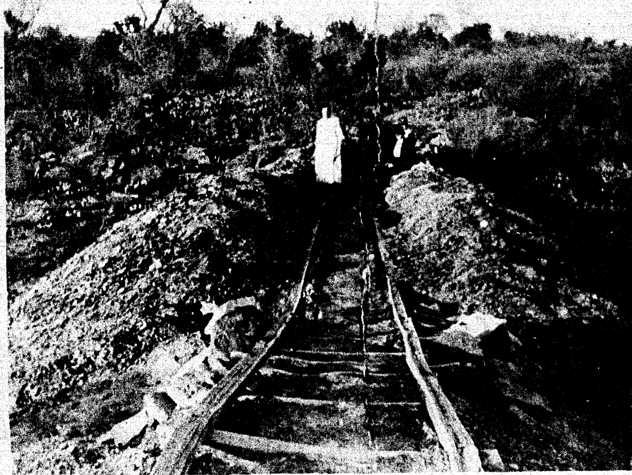
ROCKWOOD MINE— This picture, believed to have been taken about 1916, shows a portion of the wooden rails that supported the small cars that brought coal out of the Rockwood mine. According
