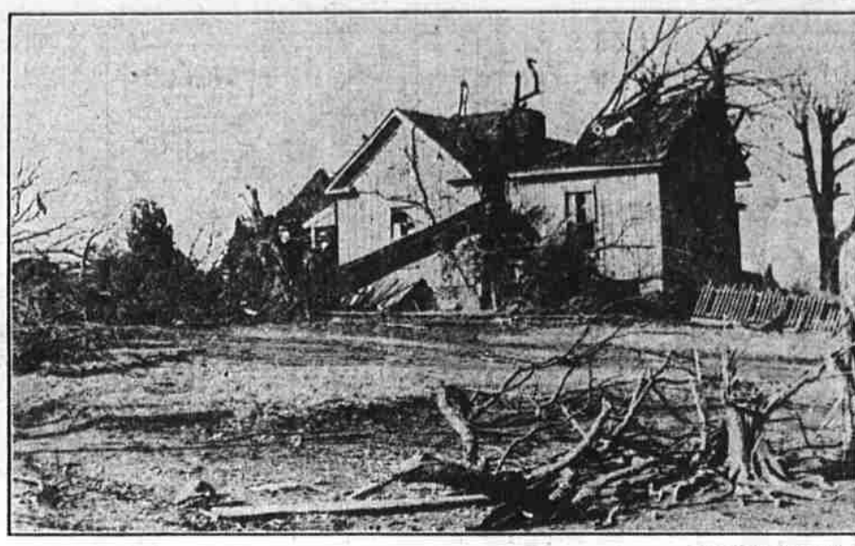
The above picture, taken in the heart of the storm area near Carterville, Ga., shows a home cut in two by a tree blown against it by fierce winds of the storm which caused heavy property damage and cost the lives of 31 Georgia persons. This was the home of T. T. Rainey, 80, from which he and his wife escaped. More than 200 persons lost their lives in five southern states.
