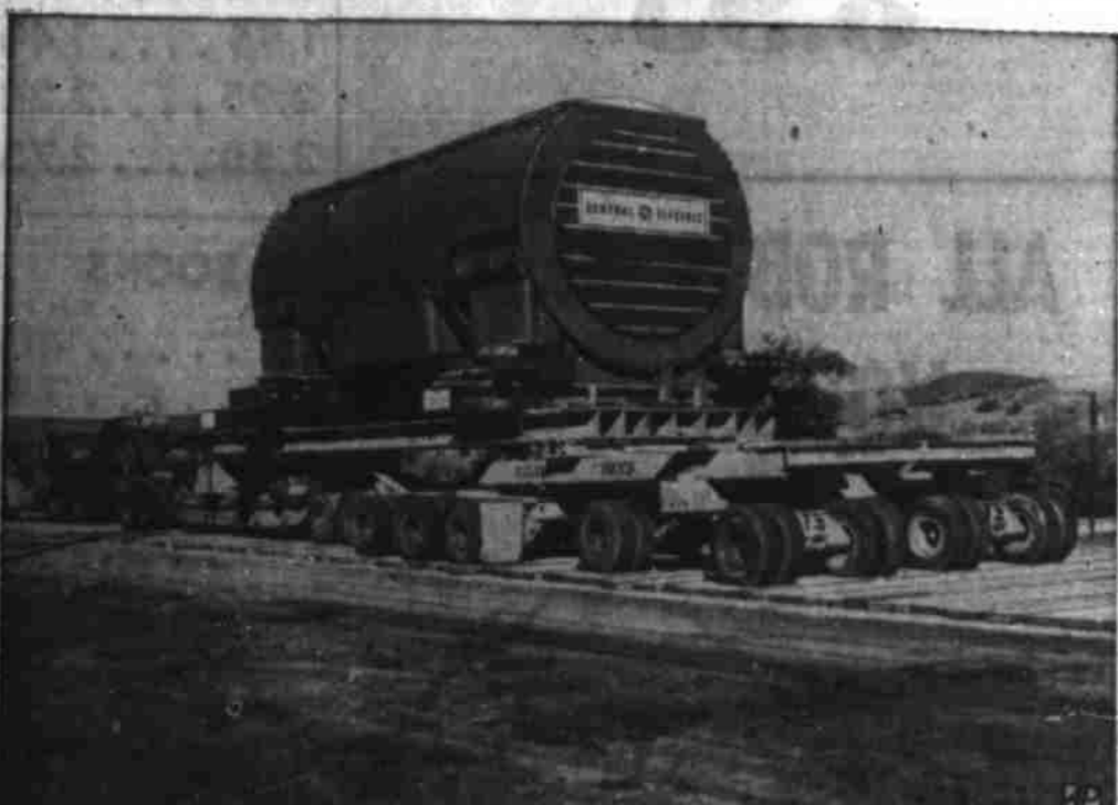
SLOWLY AND CAREFULLY —A 228-ton stator for a new power plant at Morro Bay, Cal., is moved 9.3 miles from Camp San Luis Obispo on a highway protected with planks.
