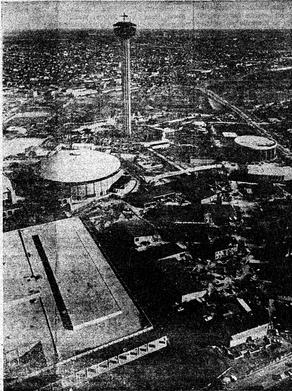
WORLD'S FAIR—HemisFair '68, only a dream a few short years ago, stands proudly in San Antonio as the last month of work continues before the April 6 opening. The $13 million civic center complex in the foreground, 622-foot Tower of the Americas in the center and the $6.75 million United States Pavilion on the right center are all prominent in the picture of the 92.6-acre showcase.
