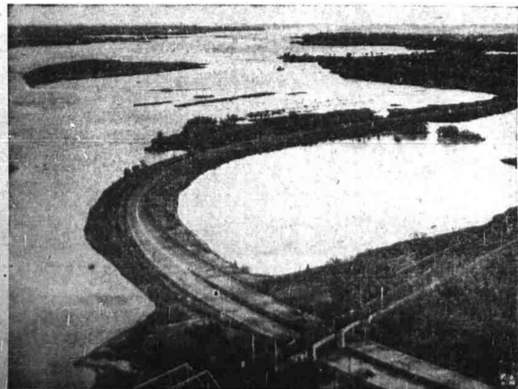
FLOWING POTOMAC RIVER marks the site for the capital's new airport for which more than $9,000,000 is available in WPA and FWA grants. The airport will comprise most of area beyond curve of Mt. Vernon Memorial highway (foreground), extending to promontory on right.
