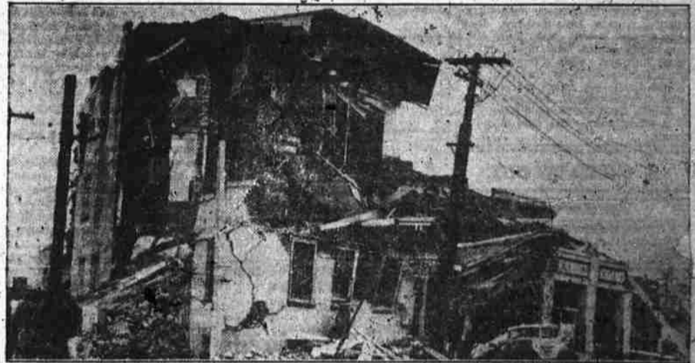
EARTHQUAKE ROCKS CALIFORNIA —One of the biggest disasters of the year befalls Southern California. An earthquake rocks Los Angeles and Long Beach and takes nearly 120 lives. Here is the wreckage of what once was a Long Beach baking company. In addition to the heavy loss of life, the quake caused a huge property damage. (Associated Press Photo).
