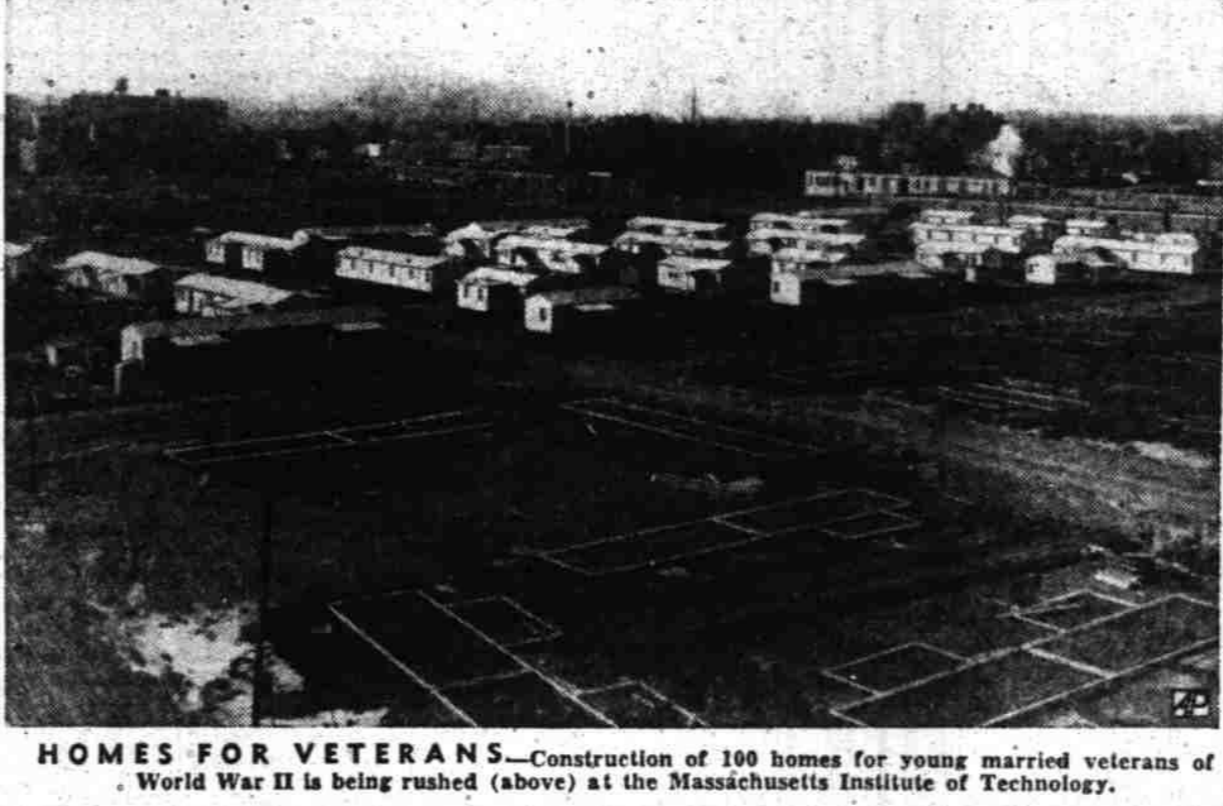
HOMES FOR VETERANS —Construction of 100 homes for young married veterans of World War II is being rushed (above) at the Massachusetts Institute of Technology.
