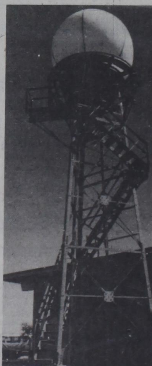
The National Weather Service uses the radar housed in this dome to help detect tornadoes and other forms of severe weather.
