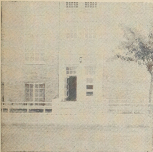
LAST WEEK'S PICTURE—West Entrance Mechanical E. Bldg.
