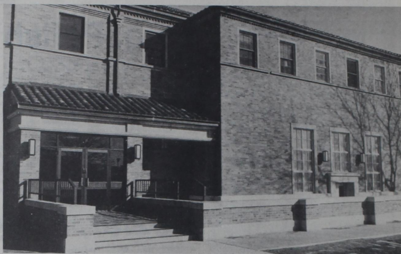
The addition to the Tech Music building is now complete
