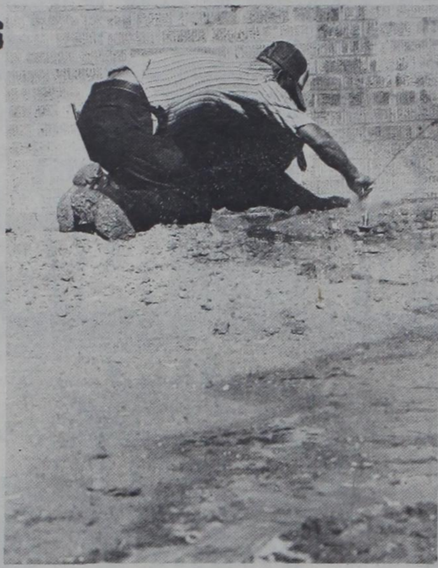
A Tech maintenance worker Thursday found out the hard way that the sprinkler he installed worked fine. The sprinkler system was being installed in front of the Math Building. (Photo by Mark Rogers).
