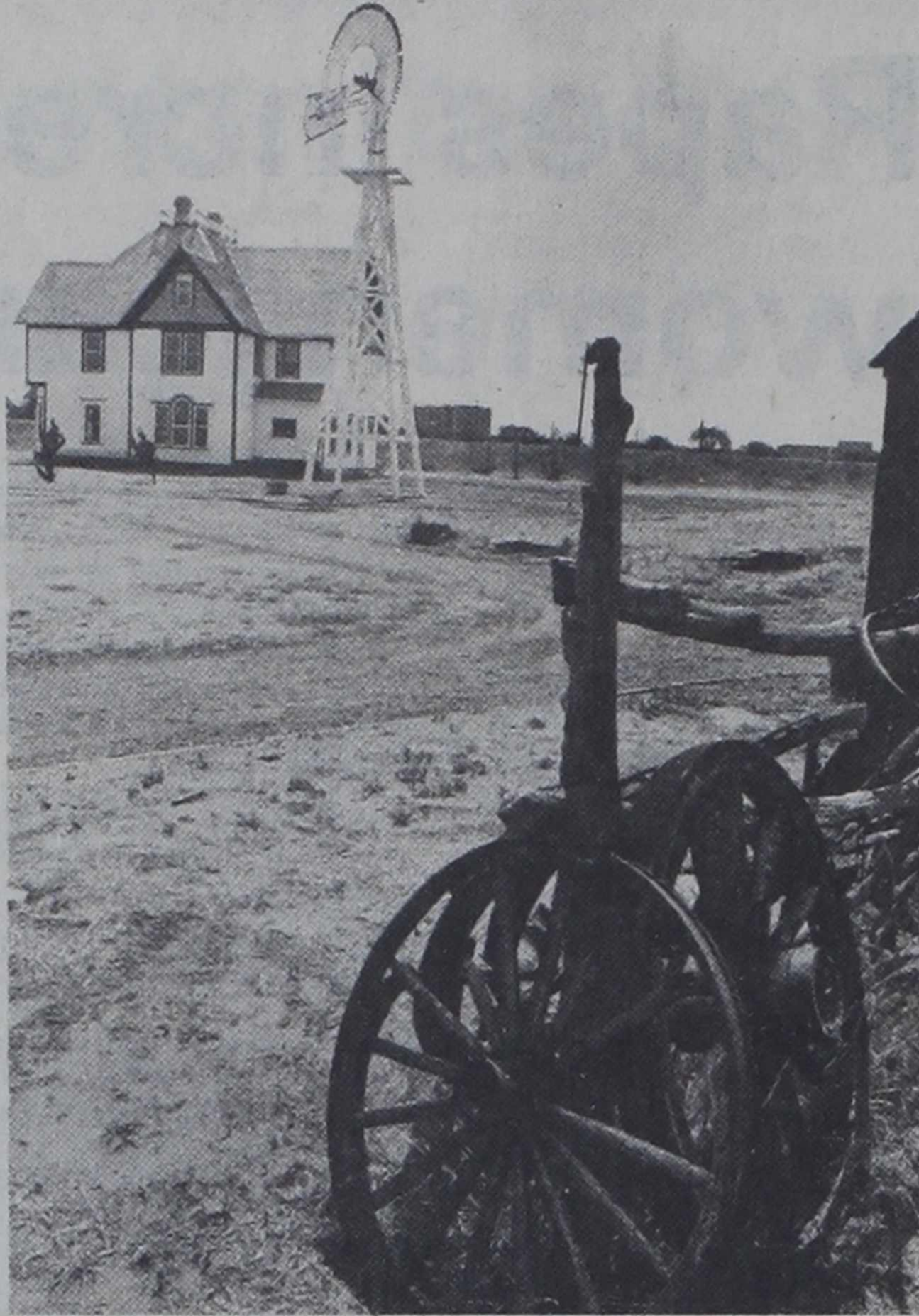
Buildings now standing at the Ranching Heritage Center were reconstructed with the structures' original materials. A new structure currently being rebuilt is stirring controversy because new materials are being used in the construction. (Photo by Max Faulkner).
