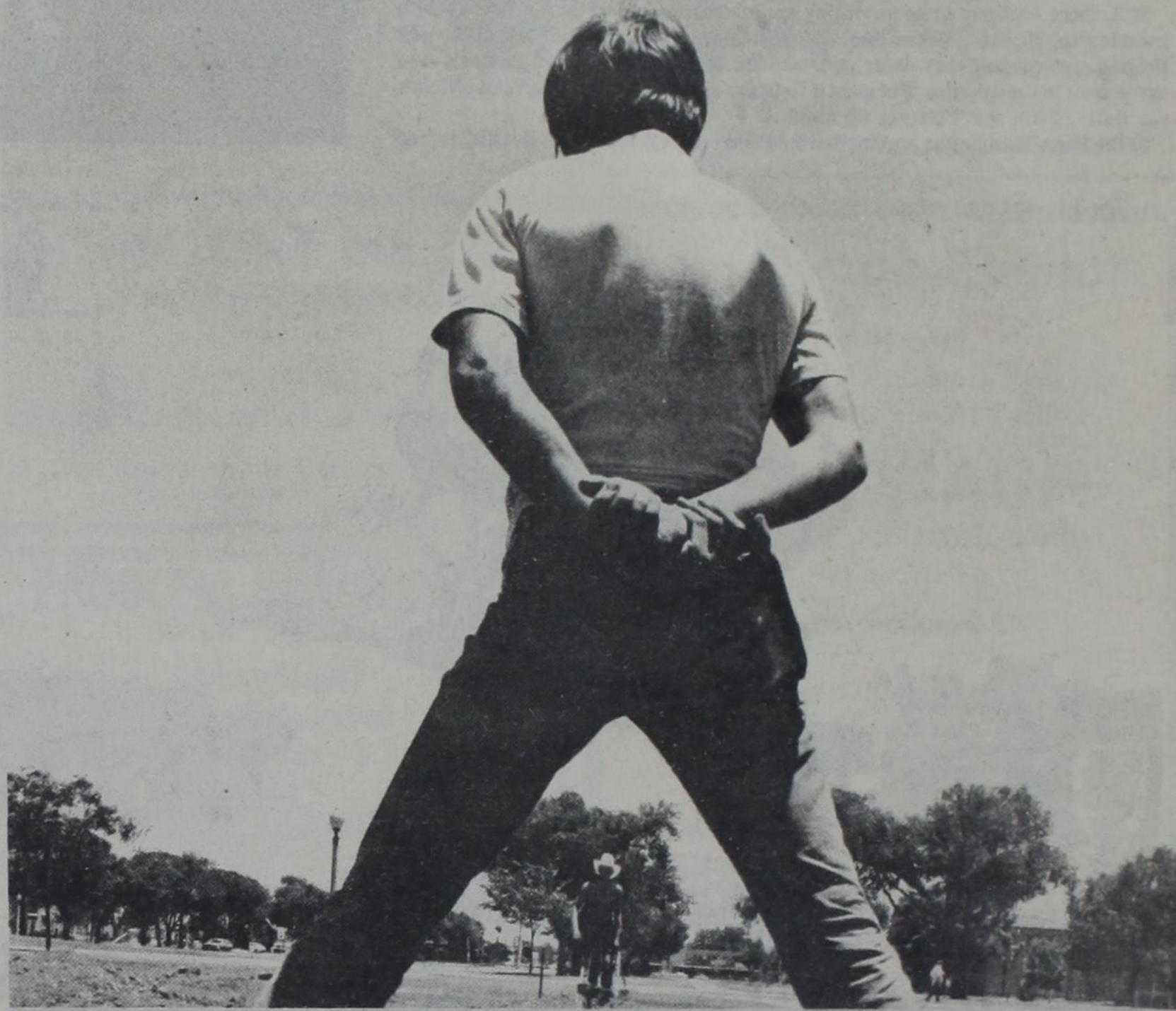
Workers on the Memorial Circle sprinkler system were digging trenches for pipes in the above 100 degree weather
