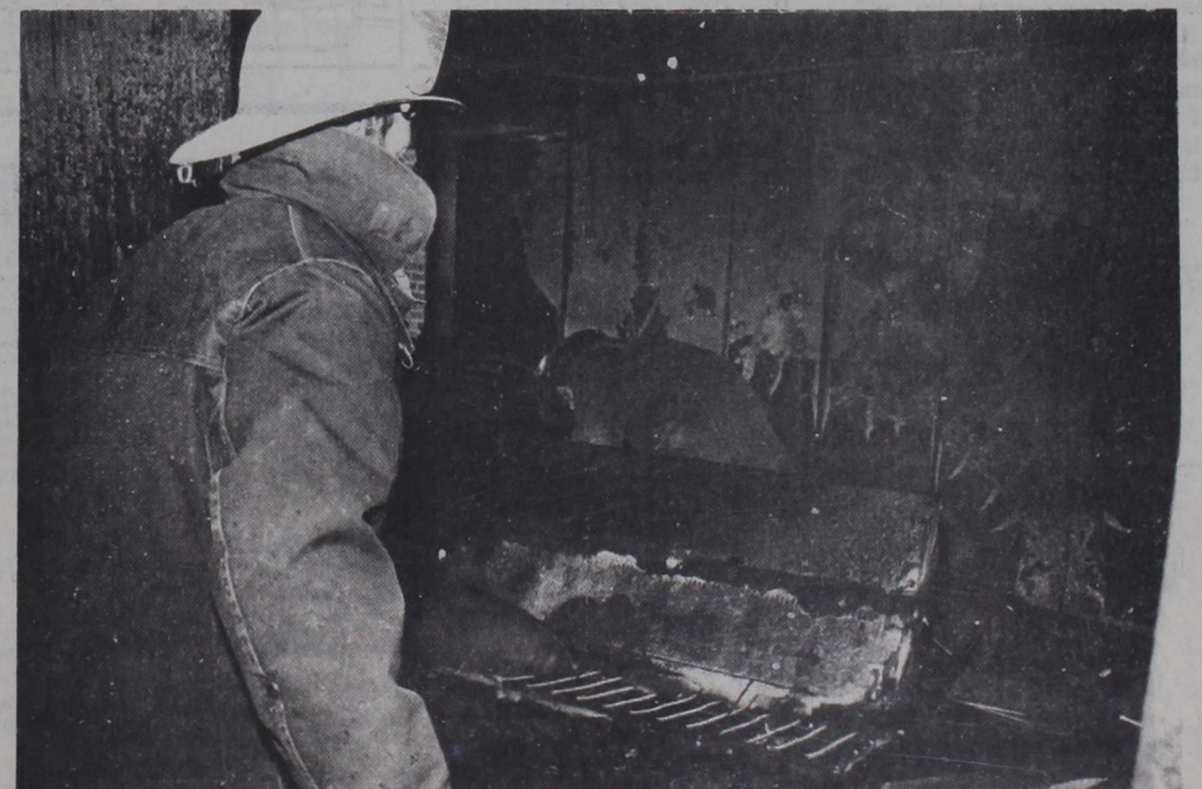
Coleman Hall damage
