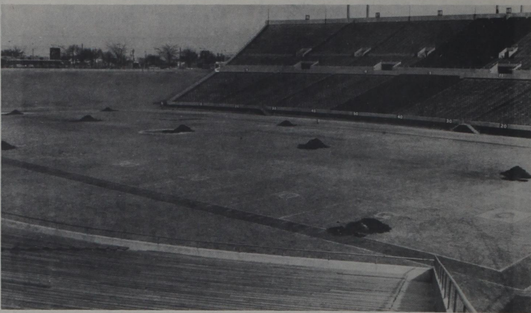
PREPARATION STARTS—The field of Jones Stadium is already changing in appearance as eleven holes have been dug out to test the soil under the turf. Astroturf is to be installed in the stadium, hopefully
