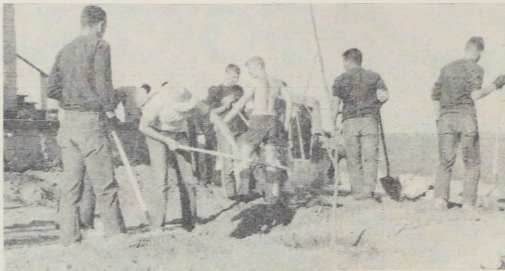
IT WAS HOT—But worthwhile as the members and pledges of Phi Delta Theta planted, hoed and moved rocks in landscaping the grounds at the South Plains Boys Ranch Saturday. It was the eighth annual Community Day project for the fraternity. —Staff Photo
