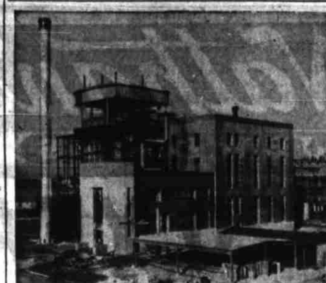
BOB POAGE PLANT—This is a general view of the new 11,500-kilowatt electricity generating plant on the Leon River, between Temple and Belton, Tex., which was christened the "Bob Poage Plant" in honor of Waco's congressman. This plant is a part of the federal rural electrification program. It eventually will be expanded to three times its present size. (AP Photo).
