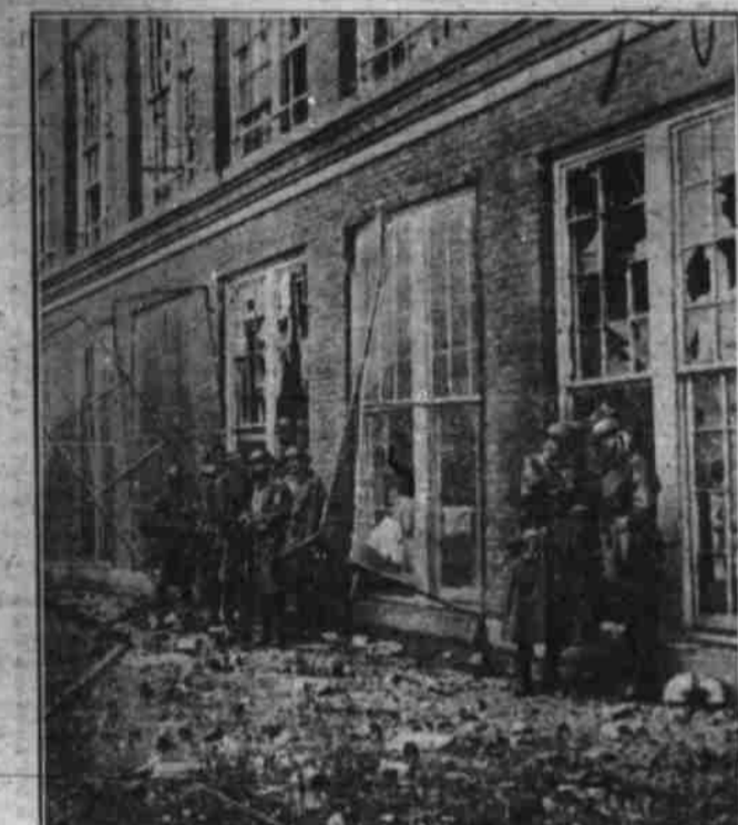
This view of one of the buildings of the Electric Auto-Lite plant at Toledo shows how countless windows were smashed during rioting there. Ohio guardsmen are shown in front of the structure. (Associated Press Photo)
