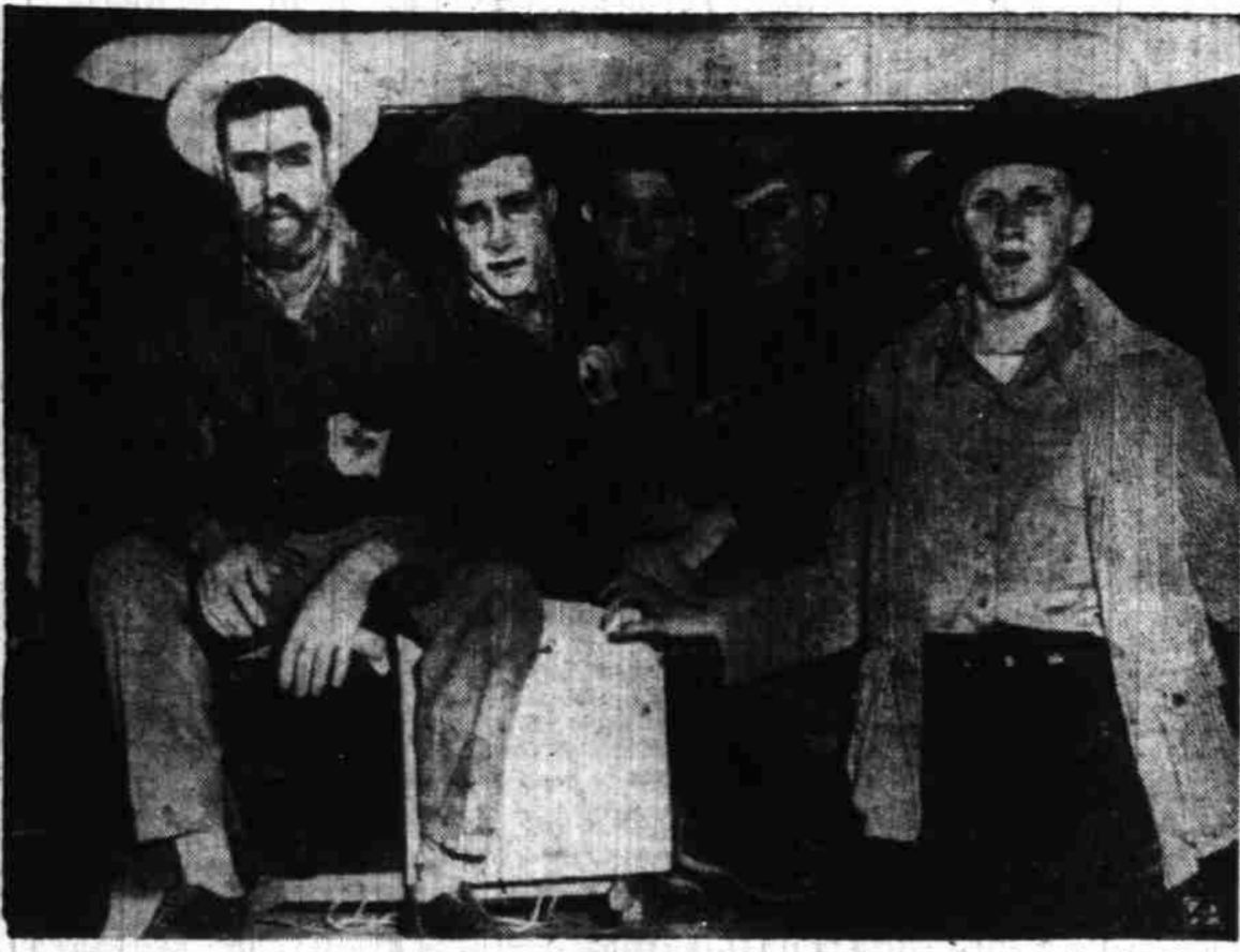
DEMOLITION SQUAD READY—Five members of a demolition squad, preparing to enter the Monsanto plant area in blasted Texas City, have their faces covered with protective ointment. All are former army demolition squad members and students of the University of Houston. (AP Wirephoto).
