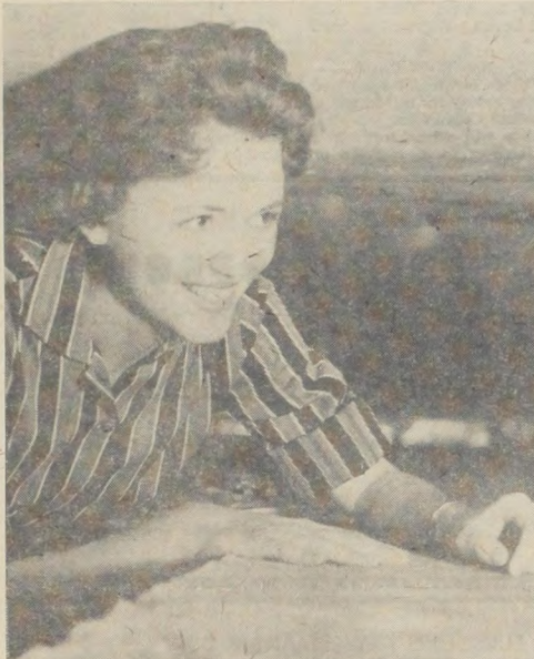
"WHAT IF IT FALLS?" comments Nita Hedleston, senior journalism major from Big Spring, as she peers beneath the giant 380-ton east roof section of Tech's new $1,000,000 classroom and office building. Raising of the slab began Friday afternoon, after several days delay due to sand in the hydraulic jacks used to lift the slabs.
