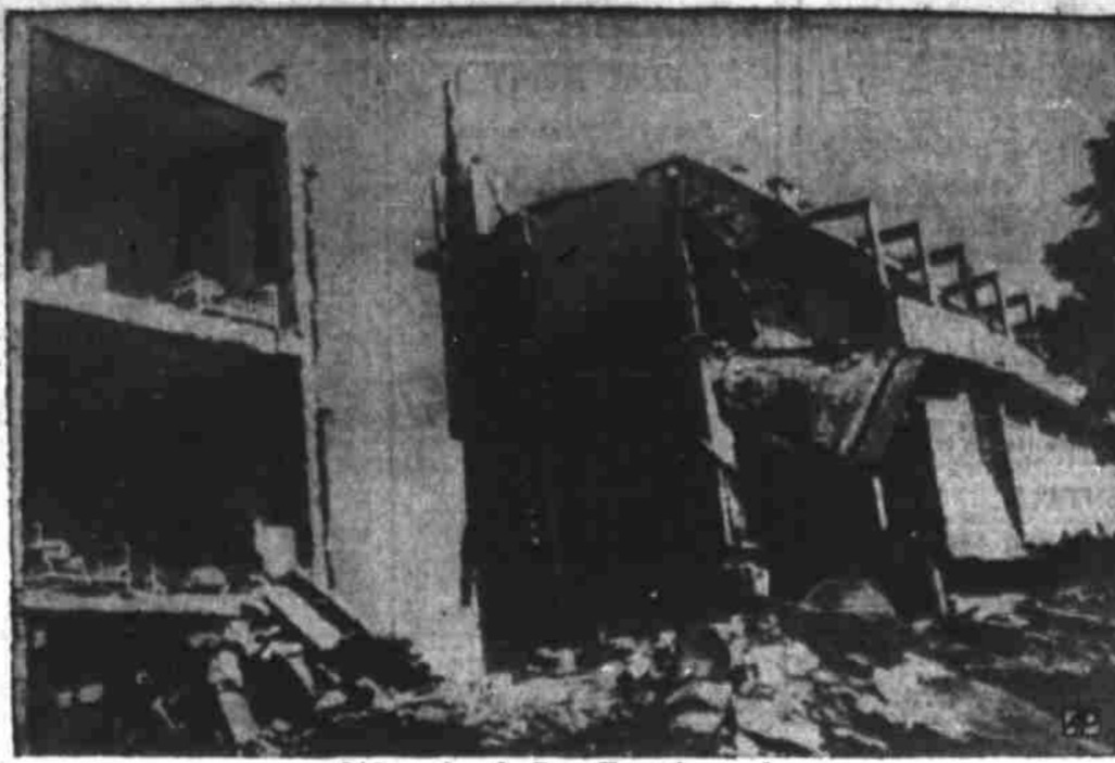
Wrecked By Earthquake
