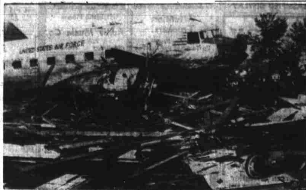
PLANE CRASHES INTO BARRACKS—An Air Force C-47 rests amid the wreckage of three wooden barracks of the Spartan School of Aeronautics after crashing into the buildings while trying to take-off at Tulsa, Oklahoma. Three janitors, each working in a different barracks, were critically injured when the plane's wing sliced through the buildings. None of the 18 men aboard the plane were hurt. (AP Wirephoto).
