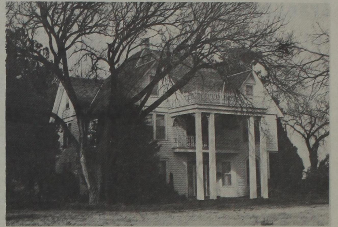
Ranch Headquarters addition
