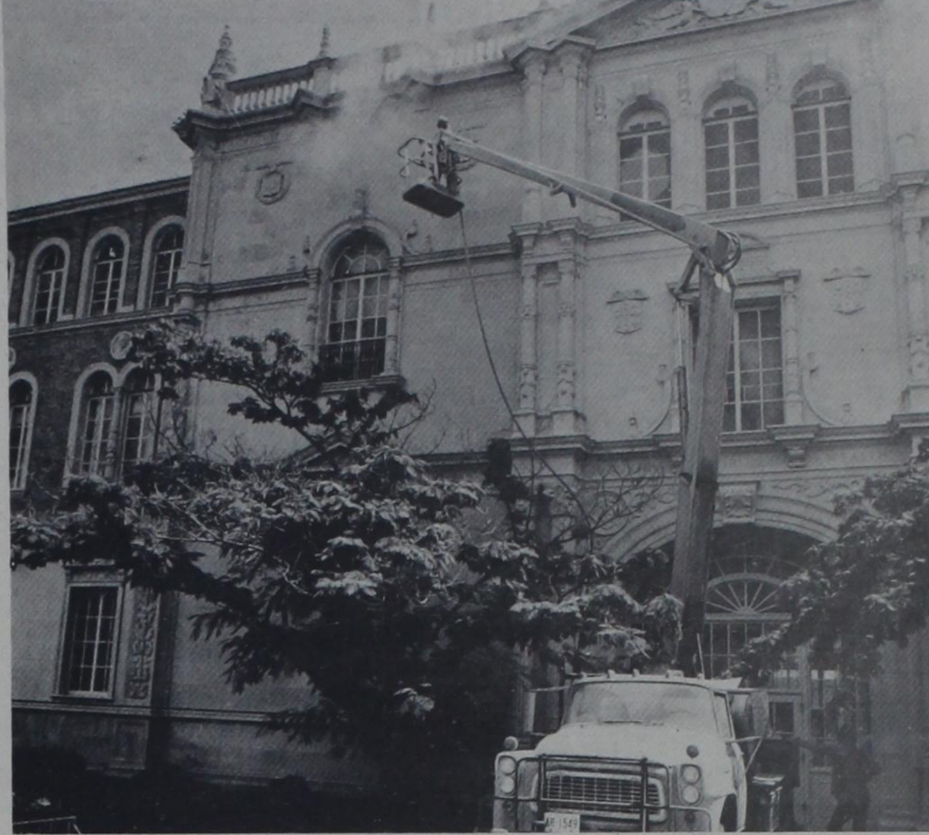
WONDER WHERE THE YELLOW WENT? — Sand, cursed though it is in West Texas, has been put to good use around the Tech campus lately as sandblasters have given the stone facades of some older buildings an almost silky white finish for the upcoming fall semester.
