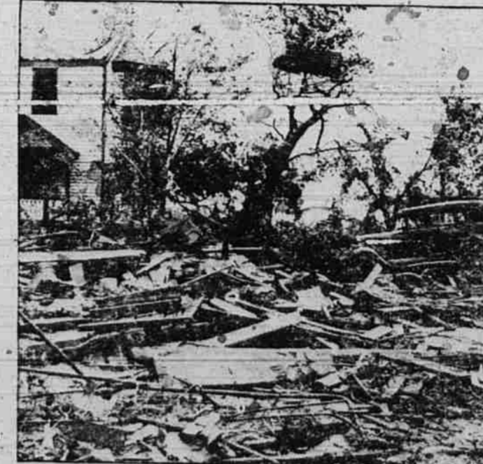
Above is a scene typical of the destruction spread by a cyclone which swept through Eureka, Mo., injuring three persons. The roof was lifted off the house at the left and the auto tossed on top of the wreckage of the garage. Part of a tin roof is wrapped about the tree in center.
