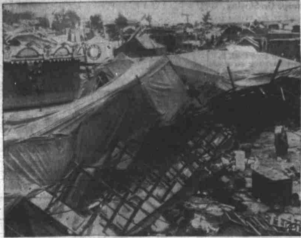
Damaged Midway At State Fair
