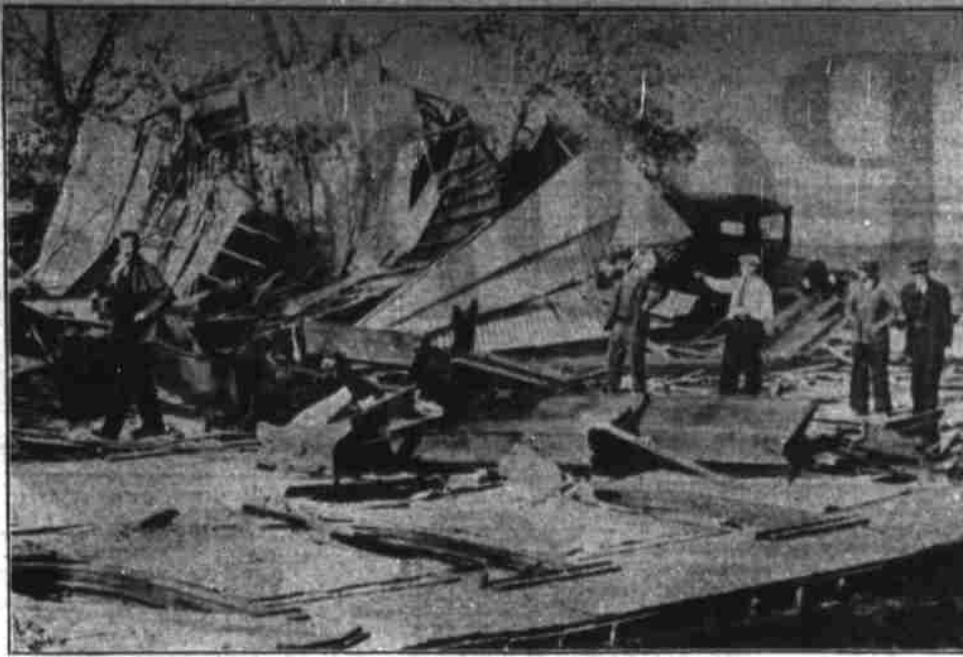
This picture shows the ruins of the Baptist church at Lake Lillian, Minn., after a tornado swept the town and injured more than a score of persons in addition to causing widespread property damage. (Associated Press Photo)
