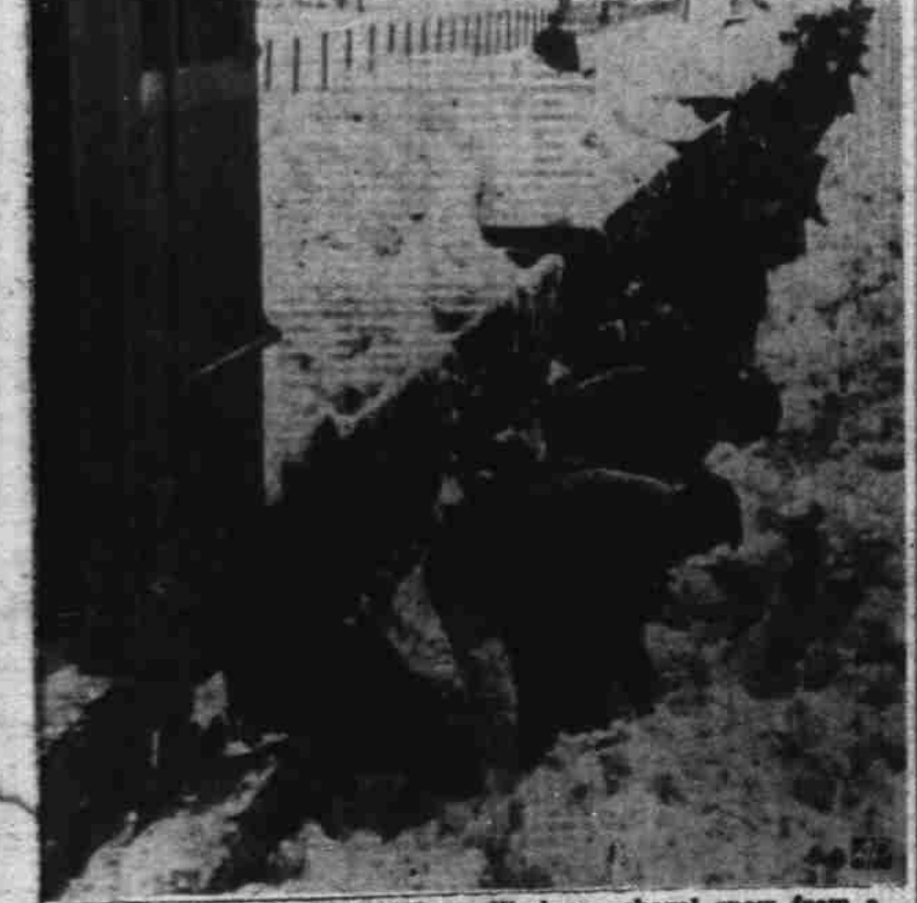
SNOW TRAIN IN ENGLAND—Workers shovel snow from a British railroad right-of-way onto coal cars which will dump it in valleys along the line. The snow is being removed to avert slides onto the tracks and flooding when a thaw comes. (AP Wirephoto).
