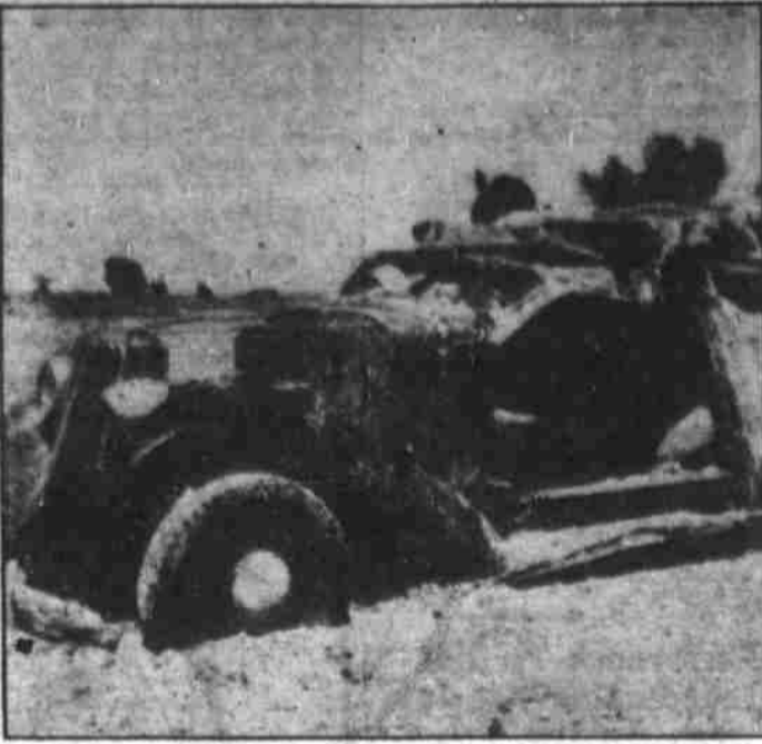
Two persons drowned, two were missing and one was rescued after this automobile plunged from the crumbling free bridge at Burkholder, Tex., into the swirling Red river during the height of the flood. Pounding waters cracked the bridge. Two other automobiles on the bridge backed off safely. (Associated Press Photo)
