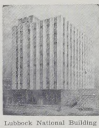
Lubbock National Building
