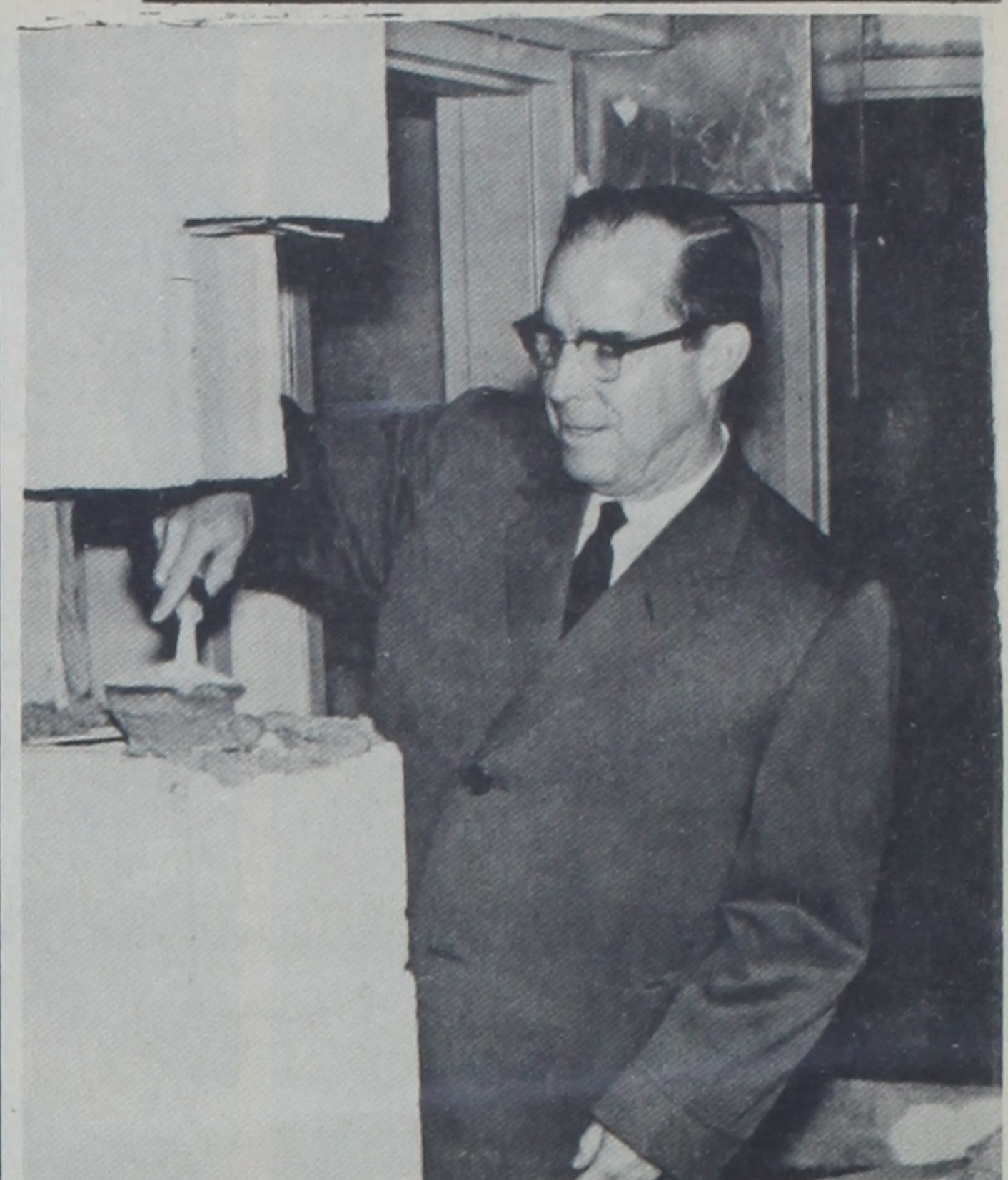
in which laborers celebrate when the top unit of a building is put in place. The other two rites are groundbreaking and dedication ceremonies. The "topping-out" was celebrated atop the new structure Thursday morning. (Staff photo by Richard Mays.)
