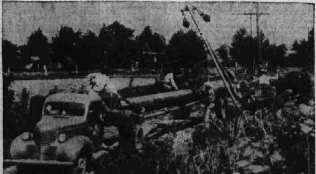
Patching The "Big Inch" —Workmen place pipe near Little Rock, Ark., on the 5-mile emergency loop which has been completed to permit resumption of flow in the "Big Inch" wartime emergency oil pipeline. The loop by-passed a break in the line caused by the flooding Arkansas river.
