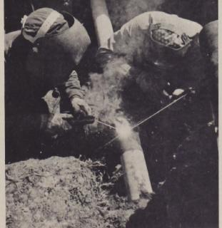
NEW GAS LINE - Tech workmen put the finishing touches on a joint of gas pipeline being installed near the Social Science Building. Olan R. Downing, director of building maintenance and utilities, said the new pipe will replace a gas line in use since Tech opened. (Staff pho-
