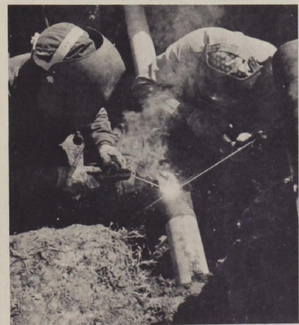
NEW GAS LINE — Tech workmen put the finishing touches on a joint of gas pipeline being installed near the Social Science Building. Olan R. Downing, director of building maintenance and utilities, said the new pipe will replace a gas line in use since Tech opened. (Staff photo by Kyle Morse)
