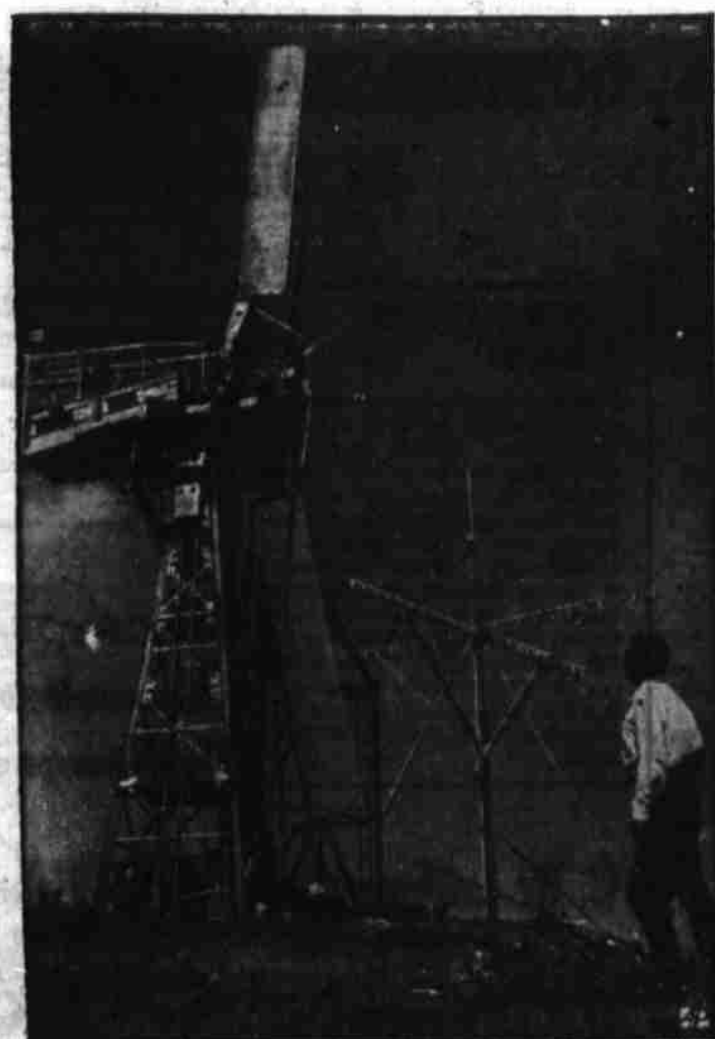
ANY WINDS TODAY? —Atop Grandpa's Knob, a 2,000-foot mountain at Castleton, Vt., this windmill whirrs around, the second of its two 22-ton, 50-foot stainless steel blades having been recently installed. The windmill is designed to generate 1,200 kilowatts of electrical power, according to its designer, Palmer Cross—Ed Putnam (above) of Boston.
