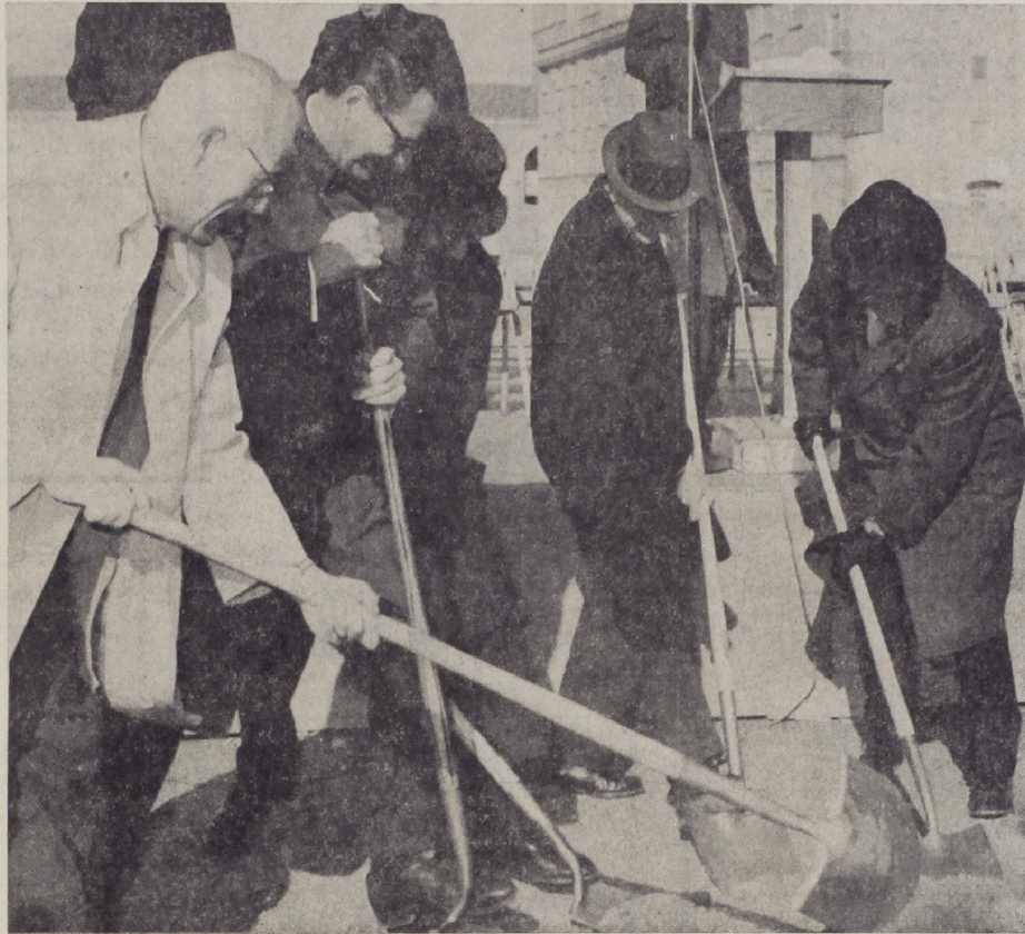
HIGH-RISE BA BUILDING — Participating in ground-breaking ceremony for the new 12-story office tower and adjacent 3-story classroom portion of the Business Administration Building are BA Dean George Heather, Tech President Grover E. Murray, Lubbock Mayor W. D. Rogers, Vice President of Business Affairs M. L. Pennington, and Tech Board Chairman Roy Furr.
