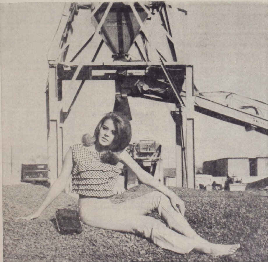
JUNIOR COED—Mary Beth Hand, attractive Fort Worth junior, enjoys Monday's springtime temperature with a view of construction on the Tech campus.
