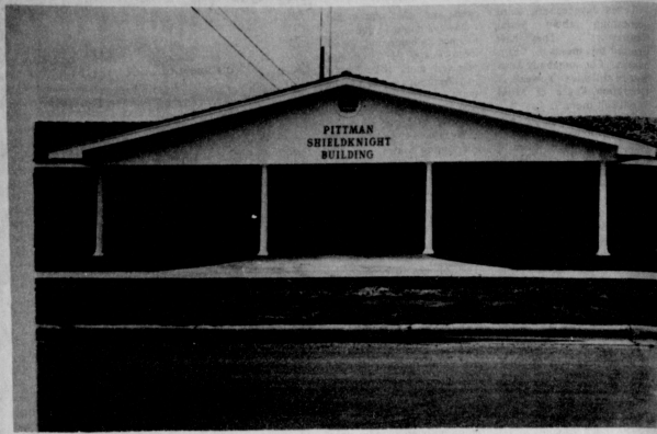
The new Pittman-Shieldknight Office Building will soon be ready for occupancy.
