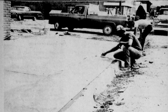
These concrete finishers were laying a new sidewalk beside the P. A. Lyon Insurance Agency downtown, Wednesday.
