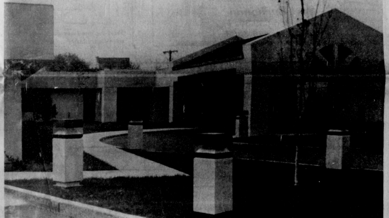
AN EXTERIOR VIEW of the newly remodeled Hansford Manor Nursing Home in Spearman. The new facility has over 33,000 square feet with a capacity to
